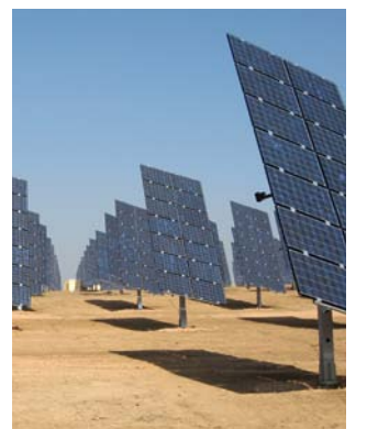
Tracked PV installation (Spain)
